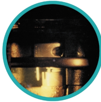
Figure 6-2. Refrigerant and oil mixture fill sight glass after week-end shutdown.
